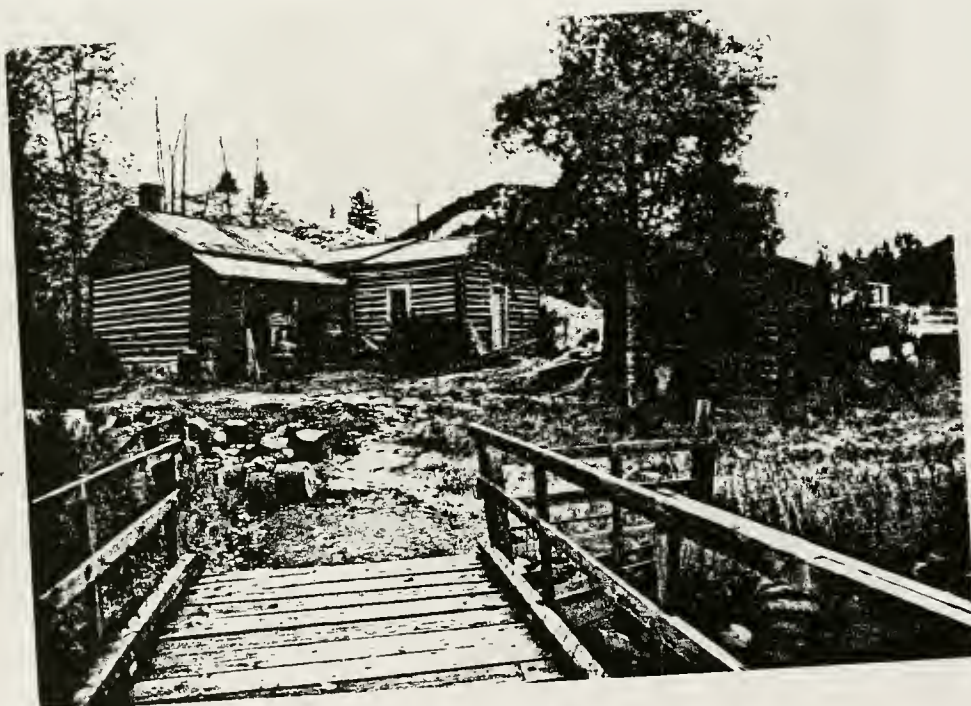
Figure 61. Structure #14, east view and structure #15.
